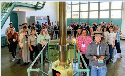
Bay-Delta Tour participants gather at the C.W. "Bill" Jones Pumping Plant, a key component of the federal Central Valley Project.
